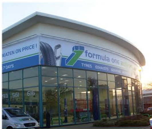
A former car showroom
